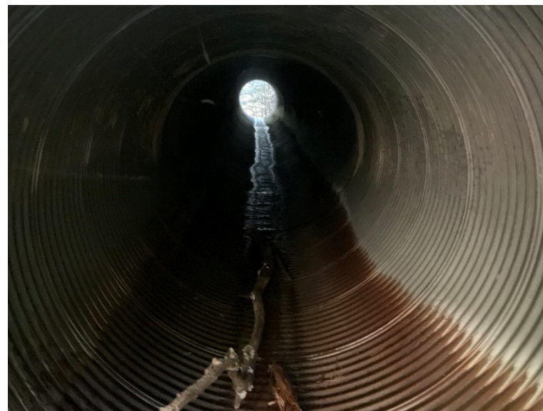
Looking Downstream Through CMP
