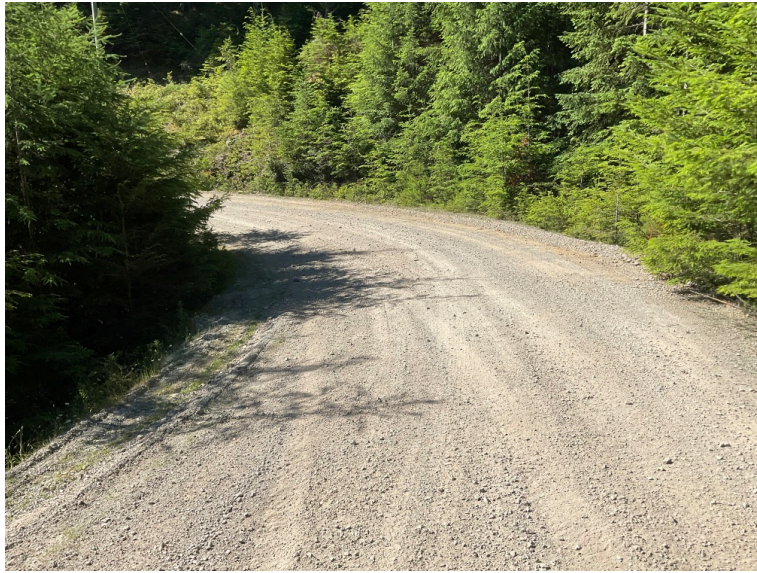
Approach from Left Bank when facing downstream
